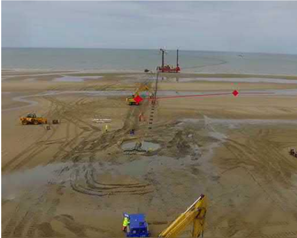
Photograph 1: Photo of cable lay across an inter-tidal area, similar to Talacre Beach, from a HDD exit pit, to jack-up cable tensioner located at approximately MLWS mark. Rollers can be seen laid across the inter-tidal with an adjacent backhoe excavator to guide the cable
