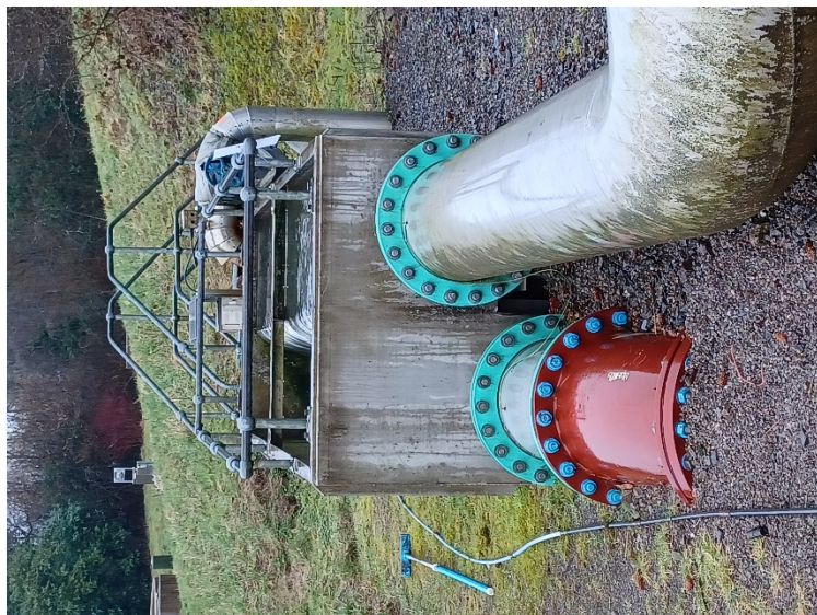
Image 1: Wastewater inlet with storm overflow weir
