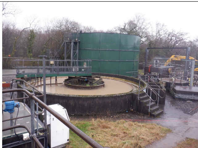
Figure 3: Primary settlement tank discoloured at the time of the visit, large green filter bed in background
