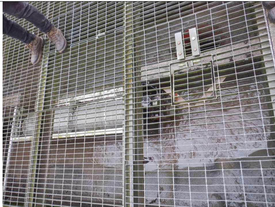
Figure 1: Inlet to works
