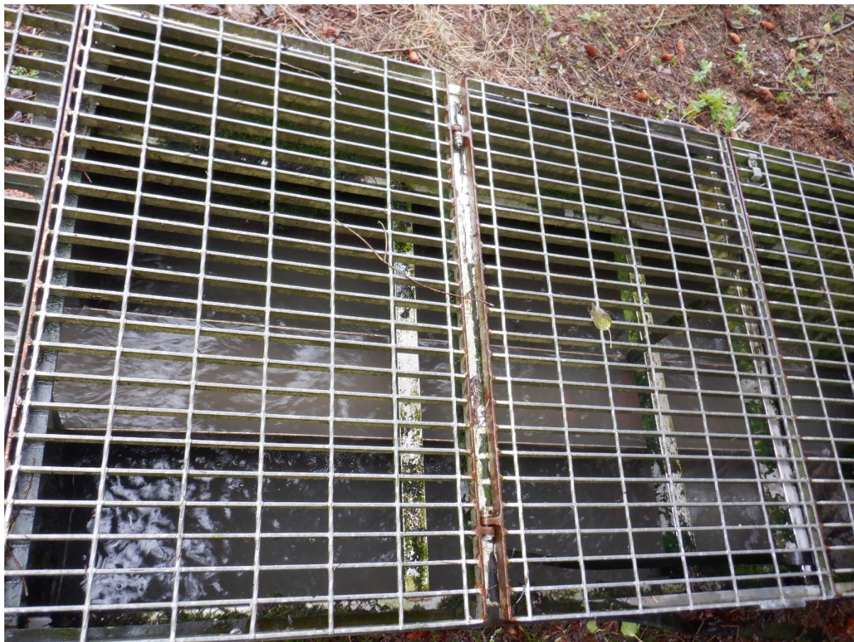
Figure 1 Storm overflow from channel and into the tank below.
