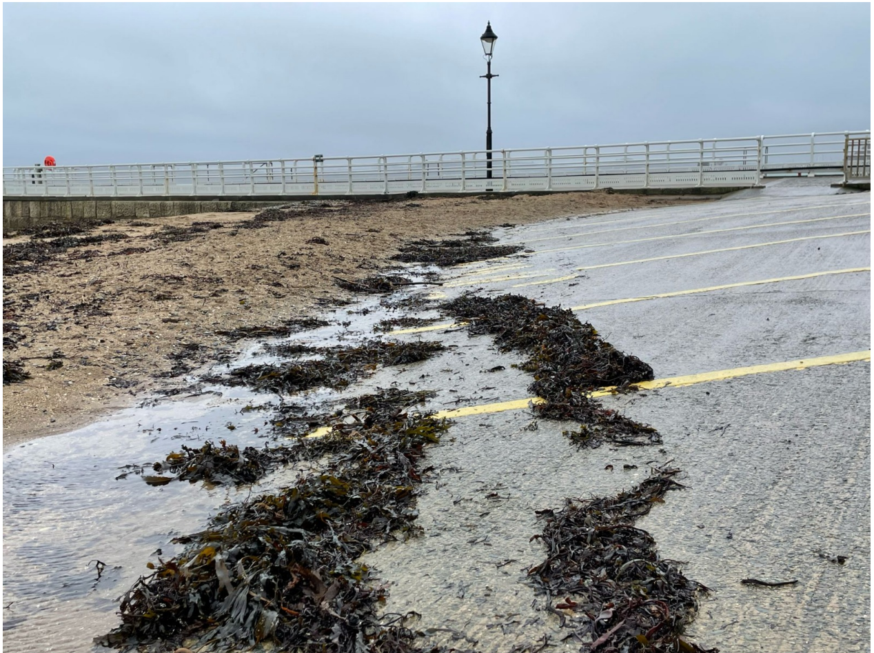
Photograph 1 - view at toe of slipway showing heaping up of beach material
