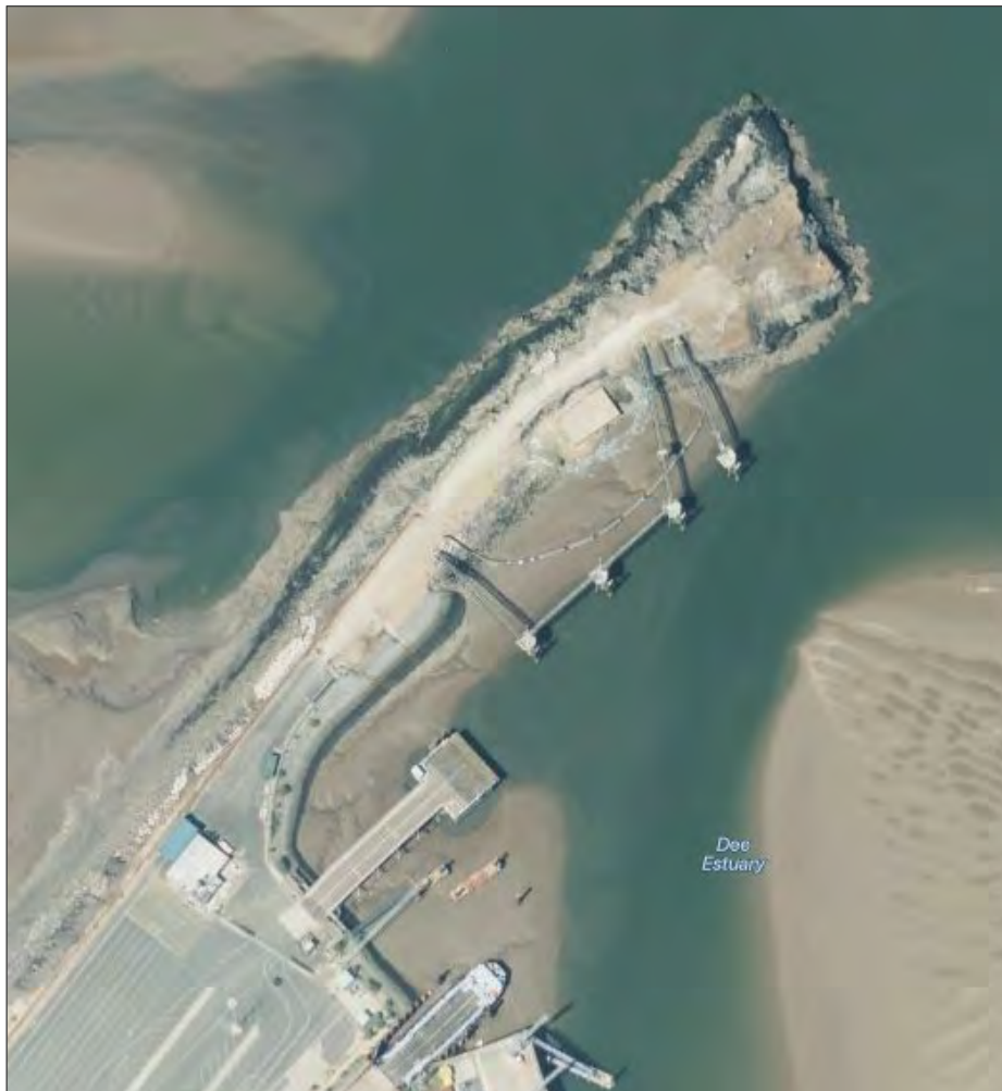
Image 3. Aerial image of the workboat re-fuelling pontoon berth, the NAABSA barge berth, and the RoRo Terminal at low water (2019)
