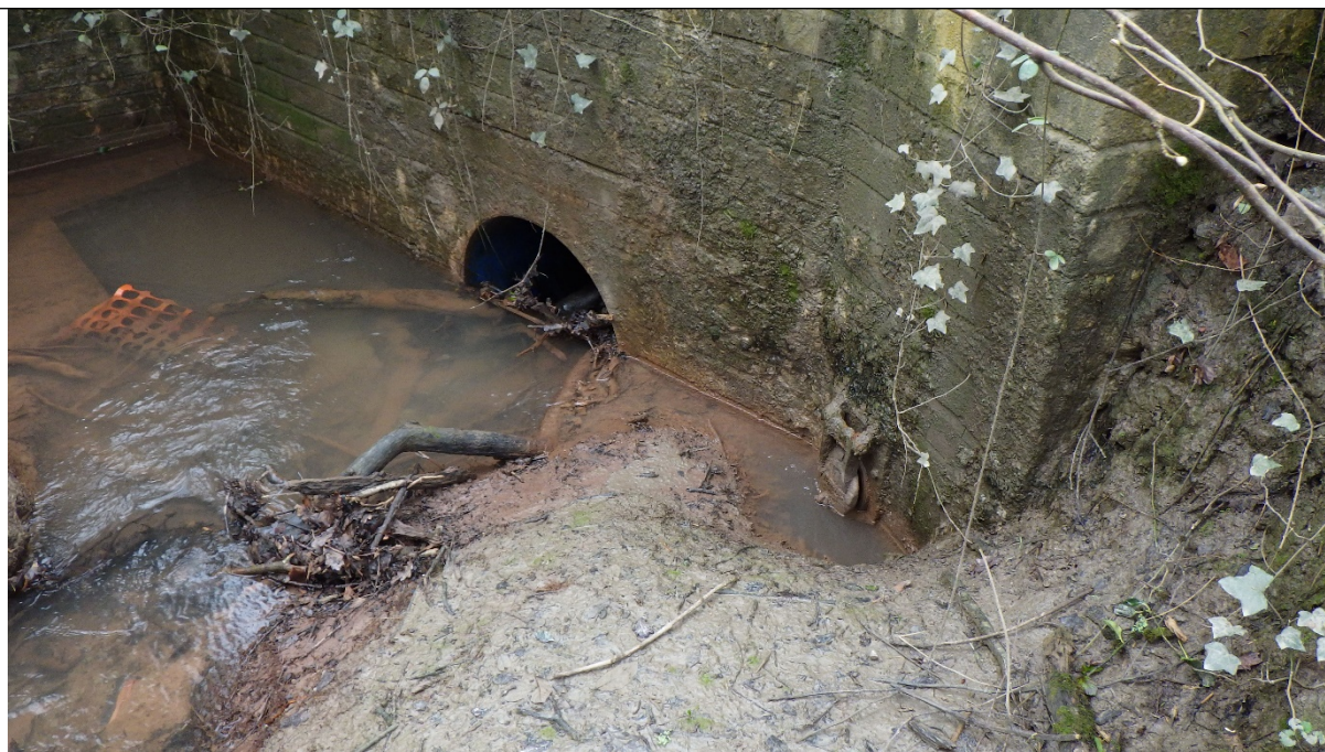
Figure 8 – Site visit photo: The discharge/sample point to the receiving watercourse. The discharge point is seen on the right hand side (small flap valve).
