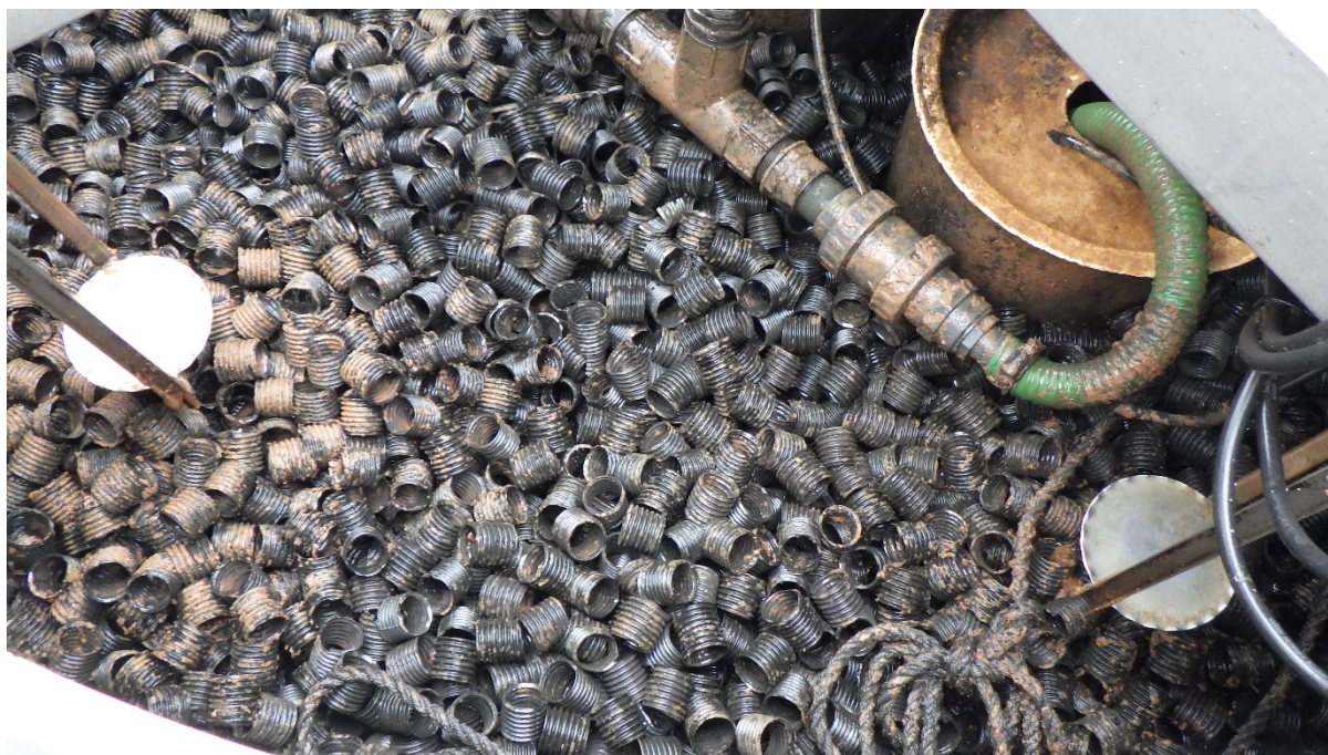
Figure 6 – Site visit photo: One of the four dispersion heads within the filtration unit. As seen, there is no excessive build-up of solid material/waste on the filtration media.
