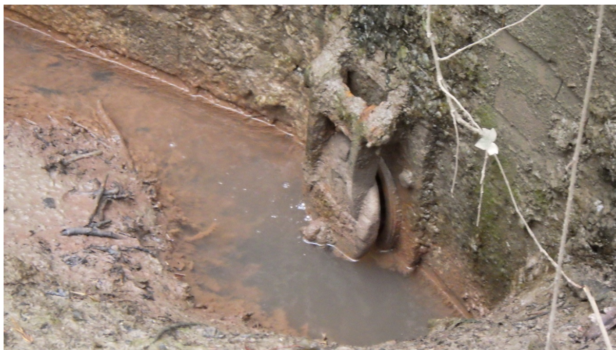
Figure 9 – Site visit photo: The discharge/sample point to the main watercourse. The pooling water appears cloudy but this is consistent with the conditions seen on the receiving watercourse.
