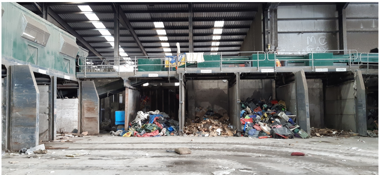
Photo 2 - View inside waste transfer station building
