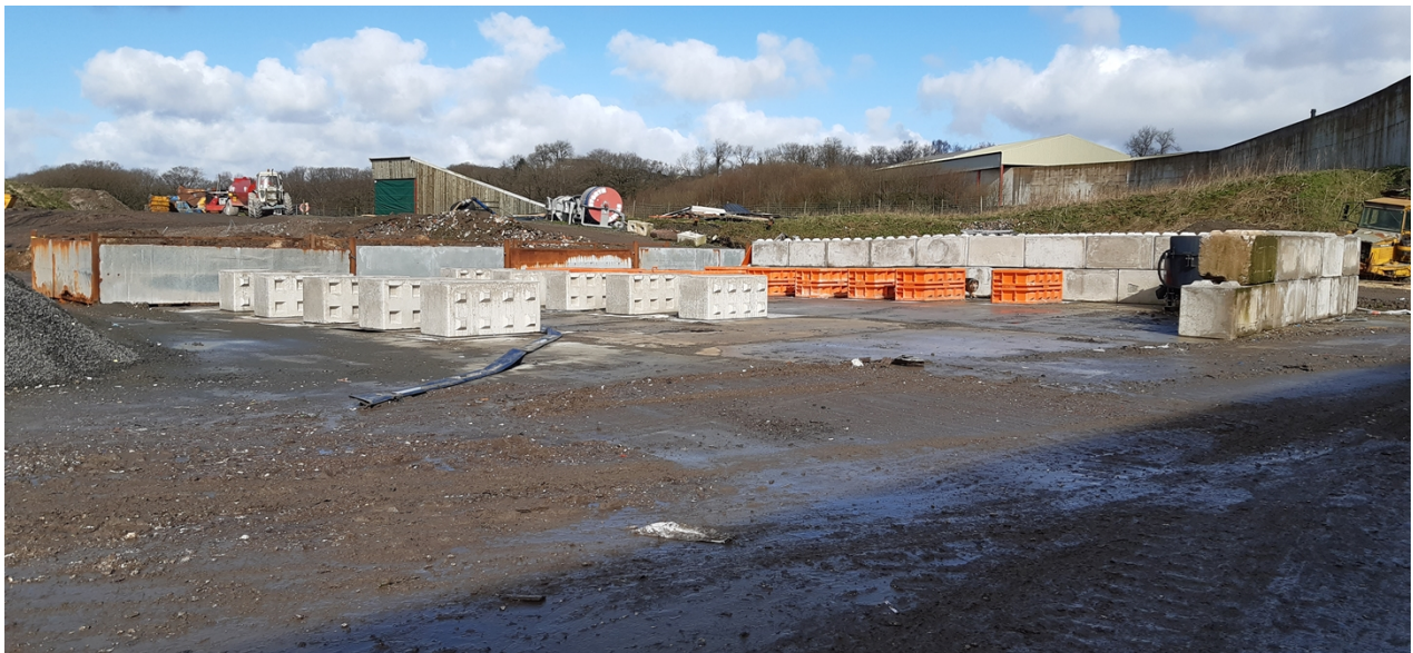
Photo 8 - Concrete 'Lego blocks' being manufactured at Bryn Recycling Ltd
