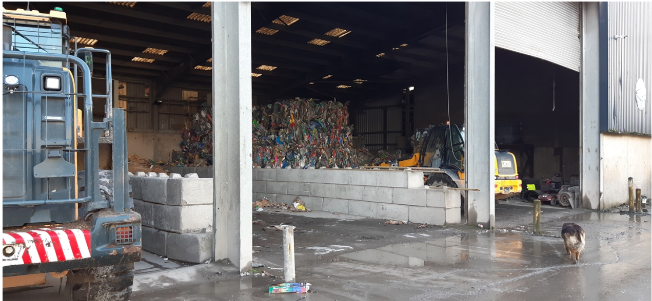
Photo 1 - View inside waste transfer station building
