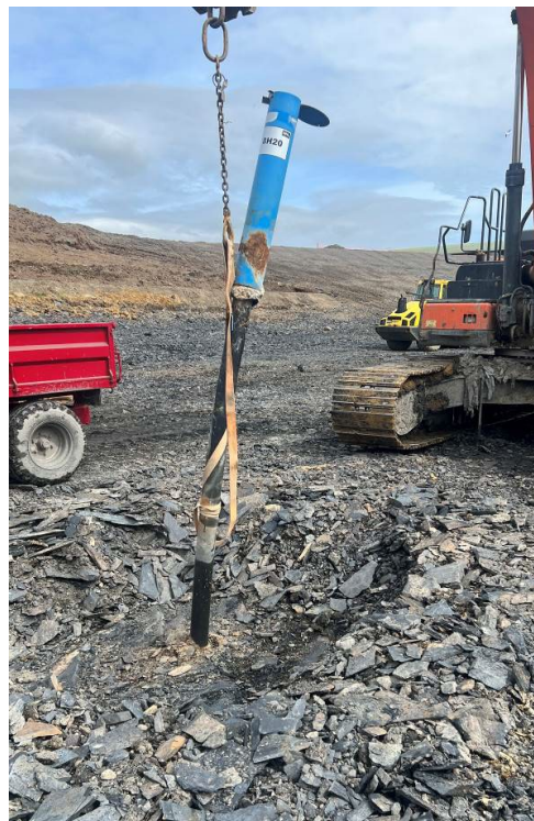
Plate 4-3 Straps Used to Withdraw Casing from Well
