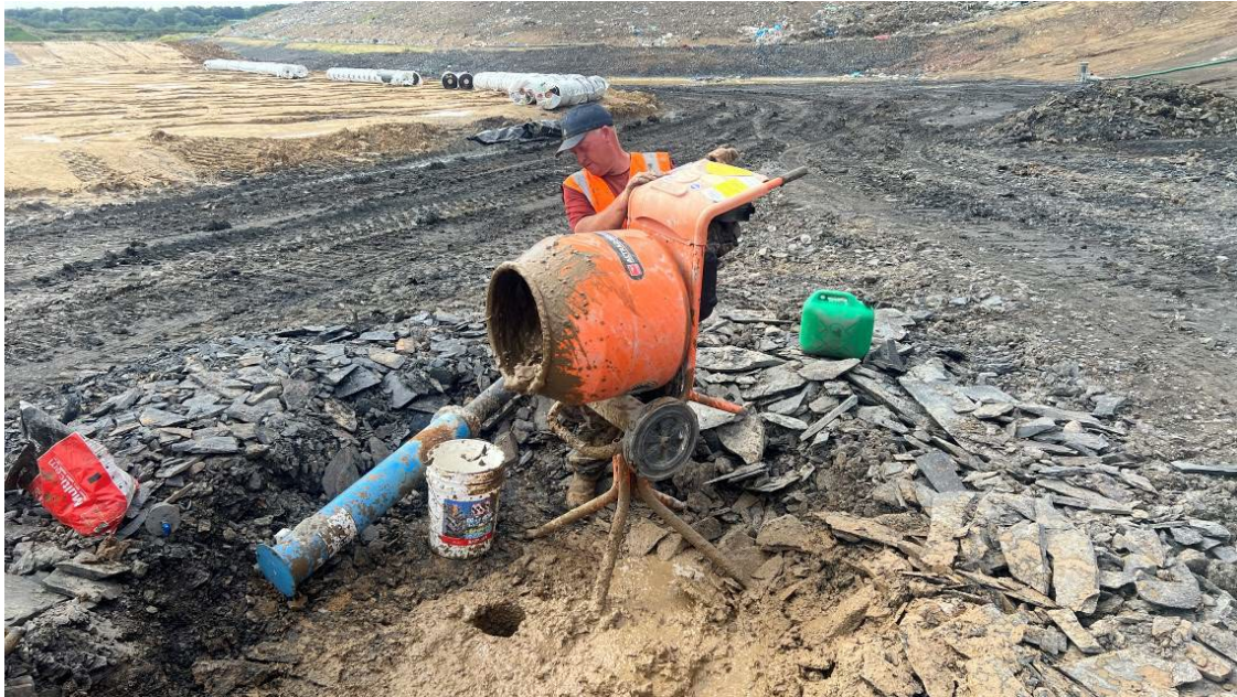
Plate 4-4 Grout Mixing
