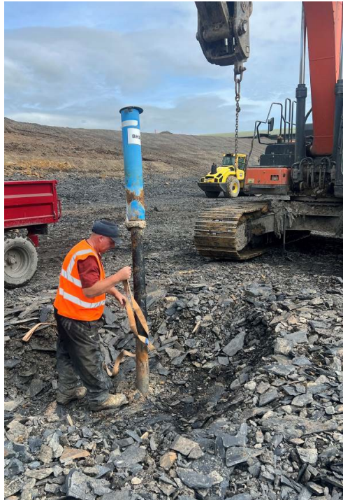
Plate 4-2 Excavation Below Formation Around Wellscreen
