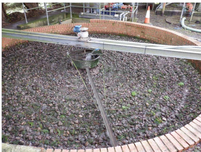
Figure 3: Filter bed
