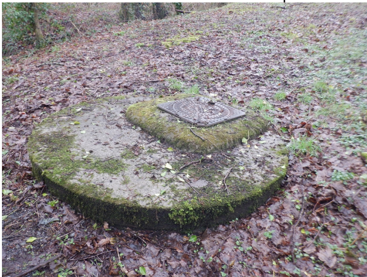
Photo showing settlement tank.
