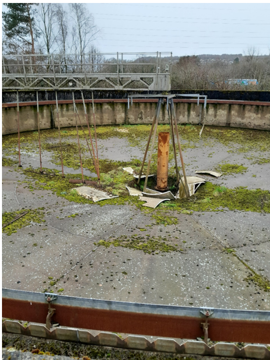
Image 1 – One of the Out of Use Storm Tanks
