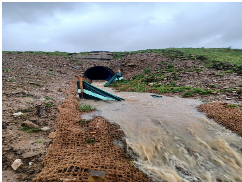
Photo 2 – discharge from pond over flocculant matting
