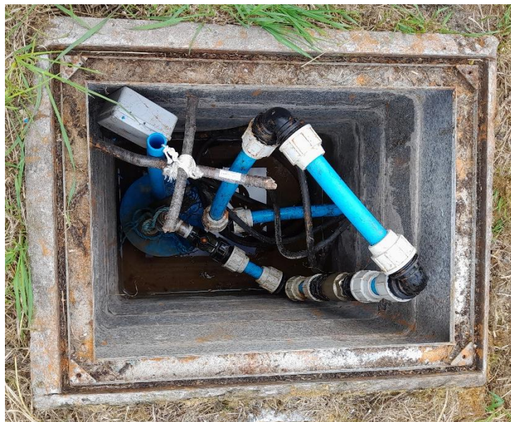
Figure 3.3 Photo of headworks at borehole BH2
