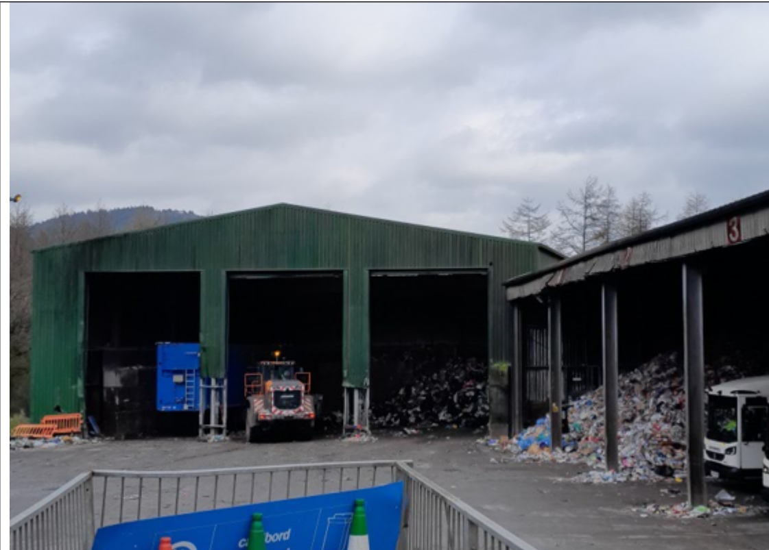
Image 1 Showing transfer station waste inside the building on an impermeable surface (note no seagulls on the roof)
