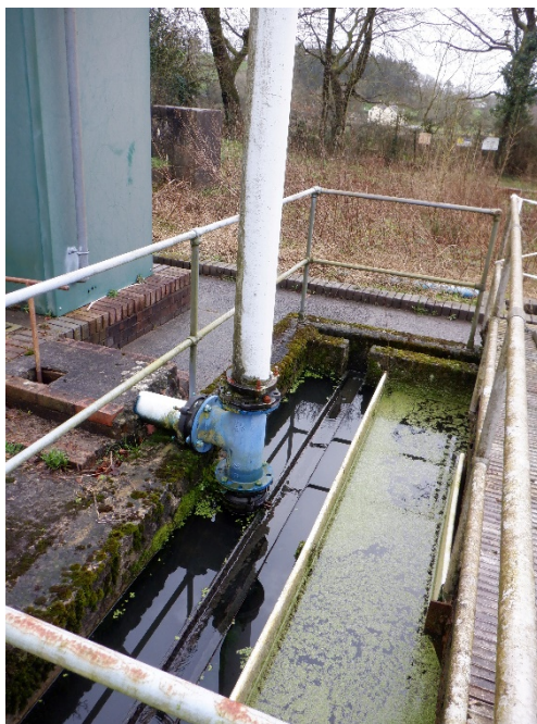
Figure 5: An image of a humus tank/final settlement tank.
