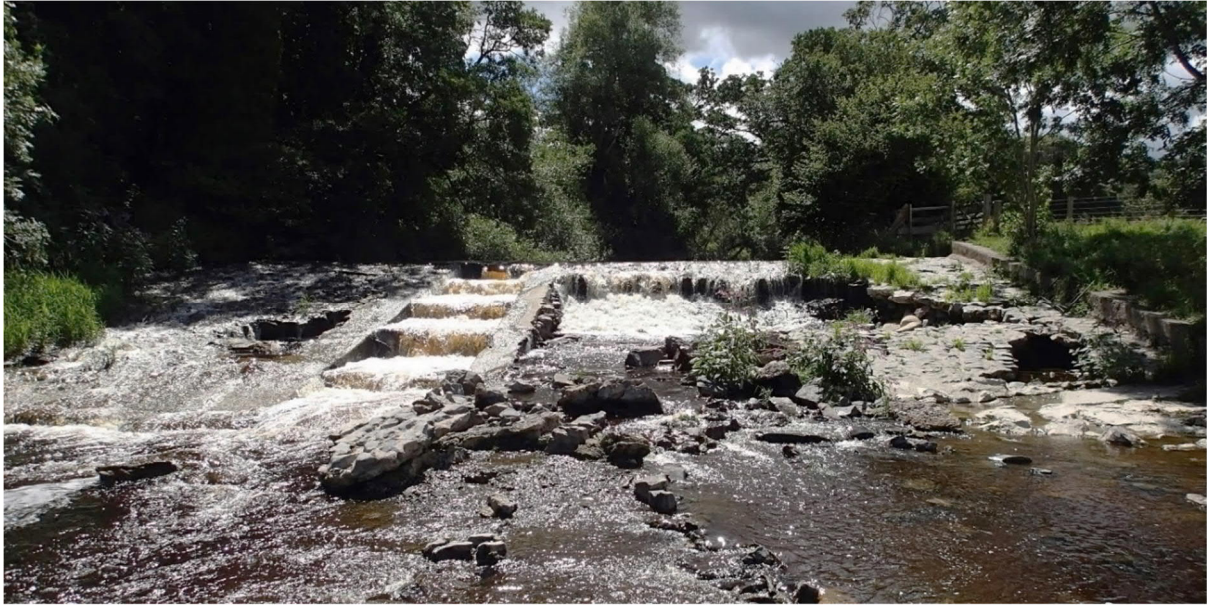
Figure 1-2 Llanfair TH weir from downstream, post collapse
