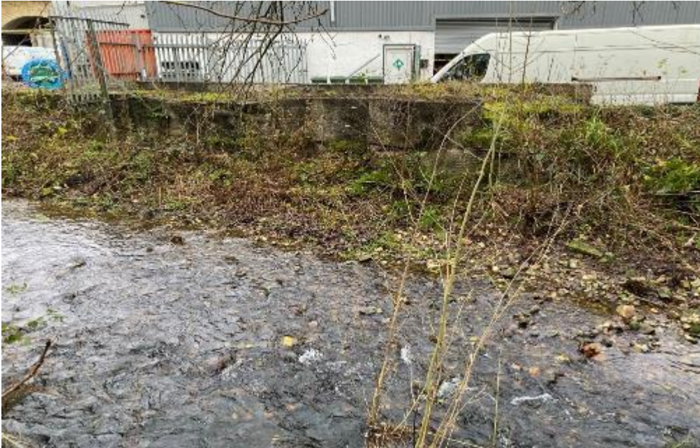
Figure 2.10. Failing gabion basket bank protection upstream of the weir at Felin Puleston adjacent to Wrexham Tyres Warehouse and the A5152 bridge
