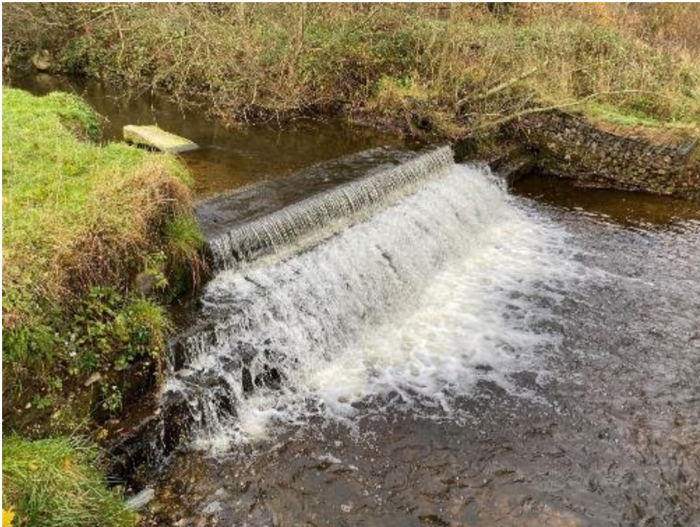
Figure 2.7. Weir structure showing three step concrete construction
