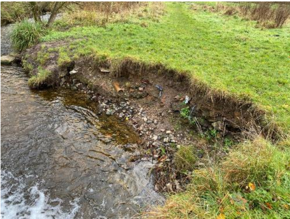
Figure 2.9. Erosion of the right bank immediately downstream of the weir structure
