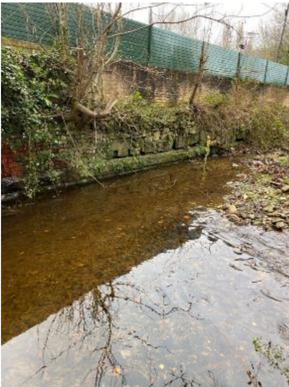
Figure 2.11. Failing walling just downstream of the footbridge
