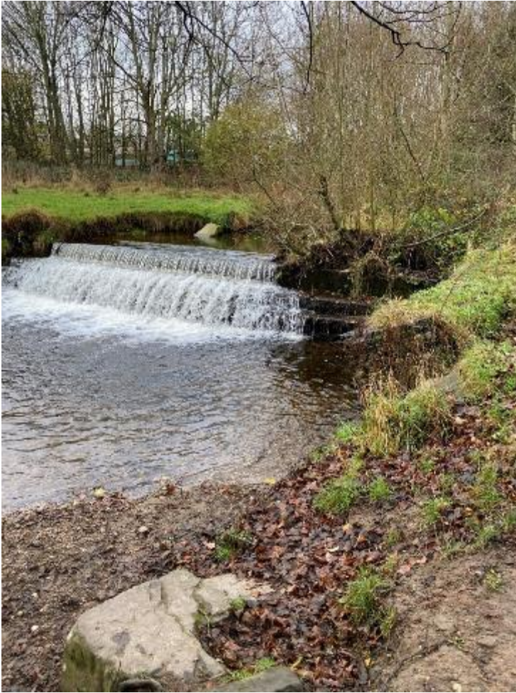
Figure 2.8. View of weir from left bank also showing leaning gabion basket repairs
