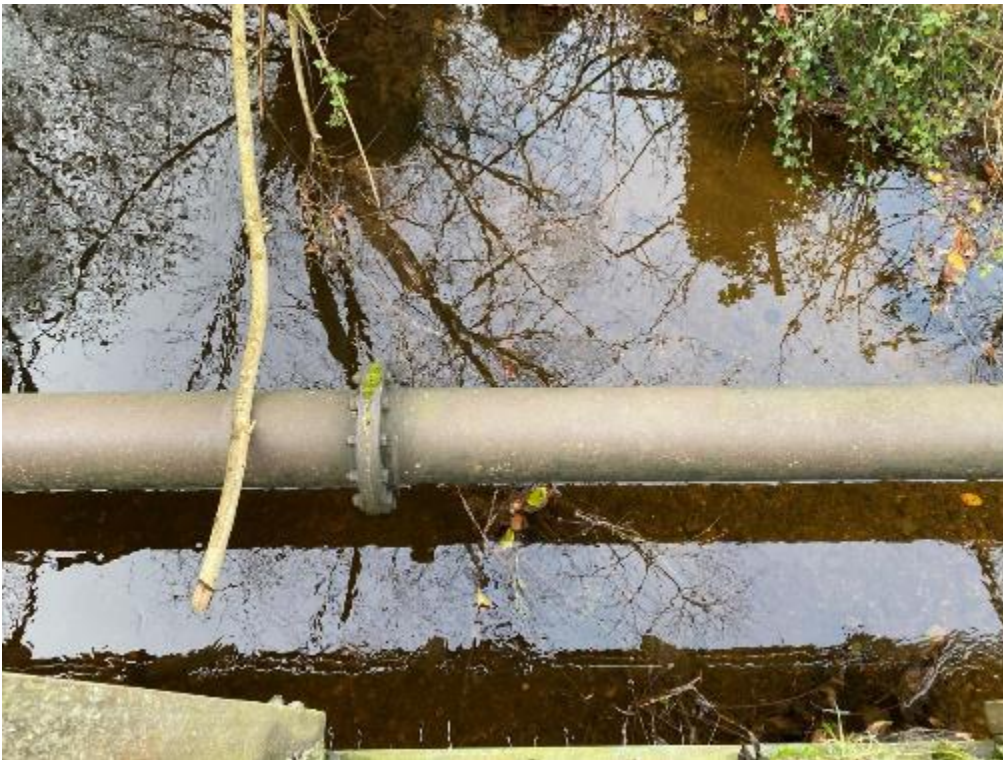
Figure 2.15. Service crossing the river along downstream face of footbridge
