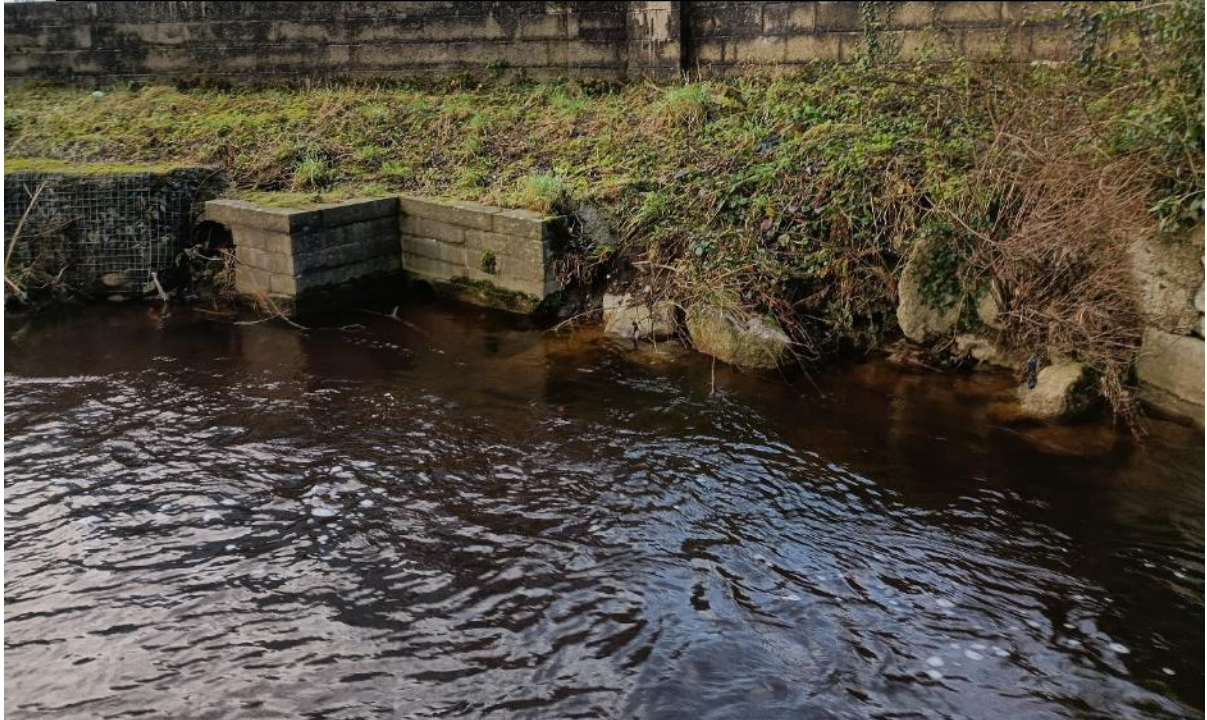
24 – LHB brickwork and gabions protecting industrial estate. RHB is not reinforced. Channel along this section narrower than downstream of weir
