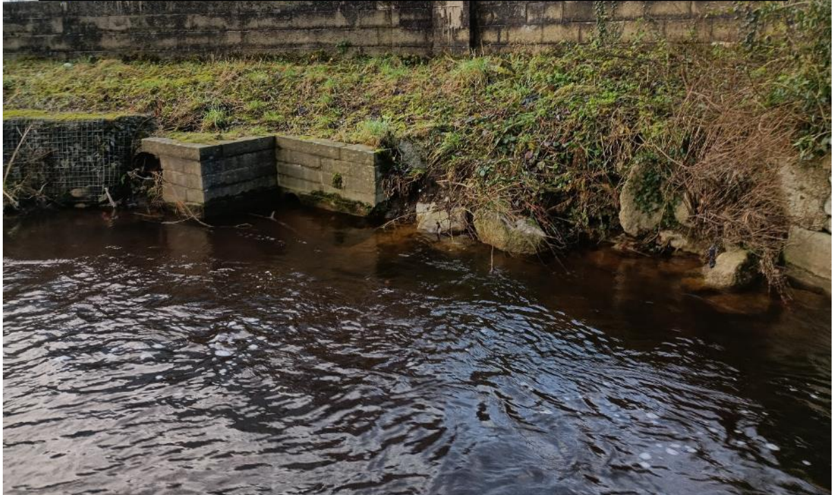
23b – SJ 32463 49318 LHB brickwork and failed stonework and gabions protecting industrial estate. River fairly deep and slow
