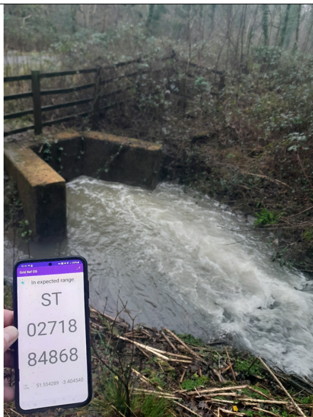
Photograph 3 – Outfall from WWTW on 23/01/2024
