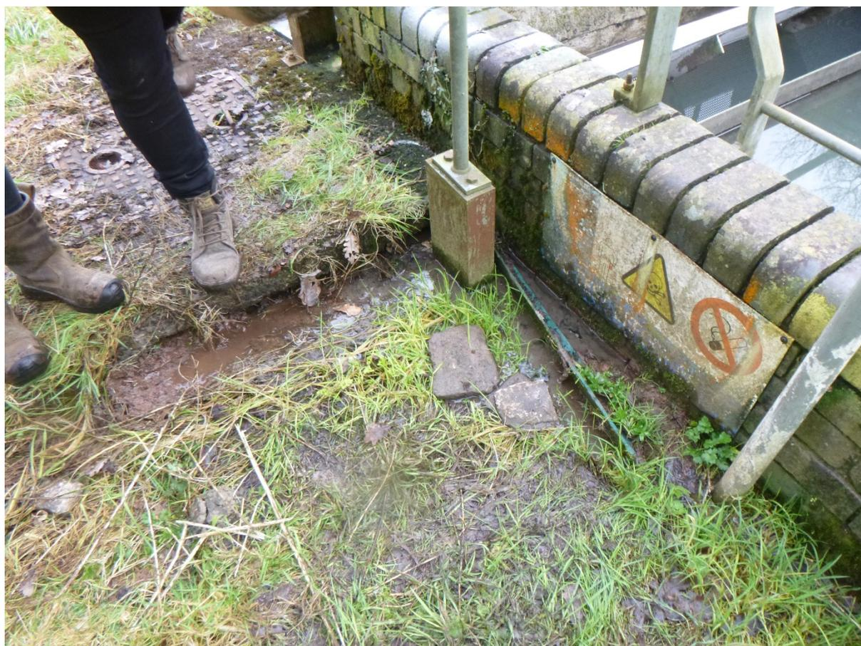
Figure 2 Leak from storm tank wall and flowing back to storm via manhole.
