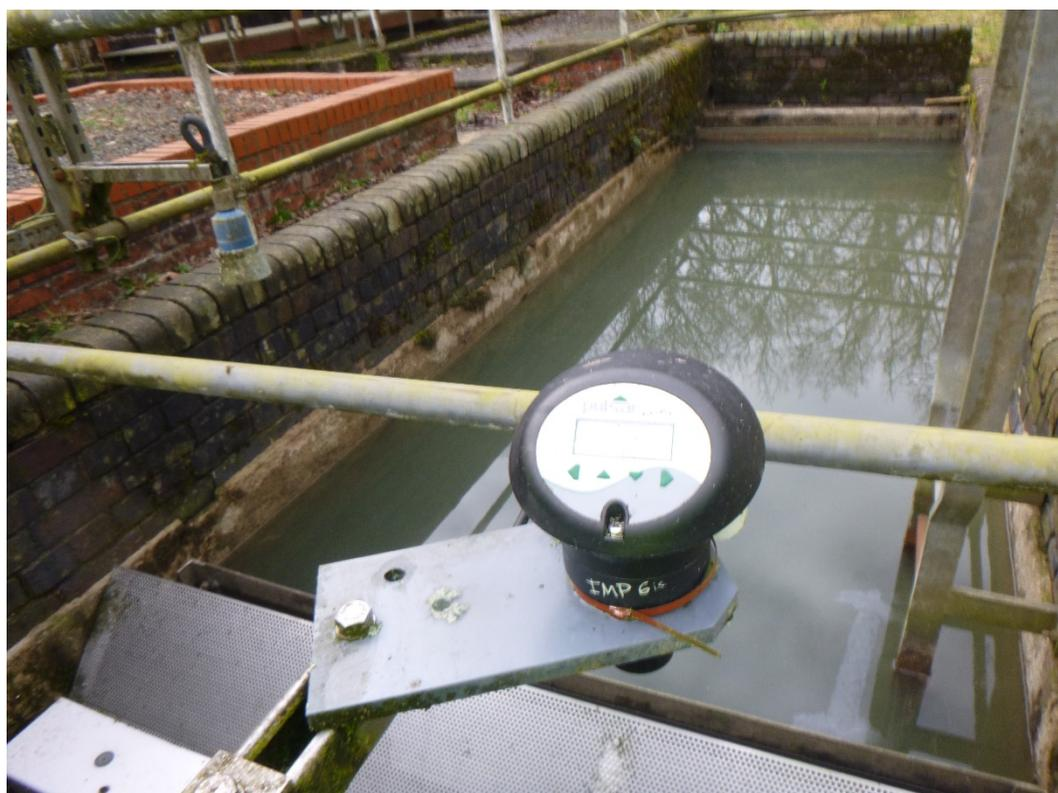
Figure 1: EDM monitor on storm tank not working.
