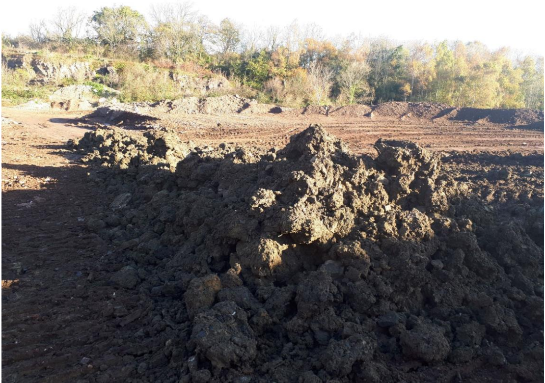
Photograph 2 – Northern sidewall showing formation for Lift 4 (surface of Lift 3) – looking east. Vegetation to be removed prior to barrier construction
