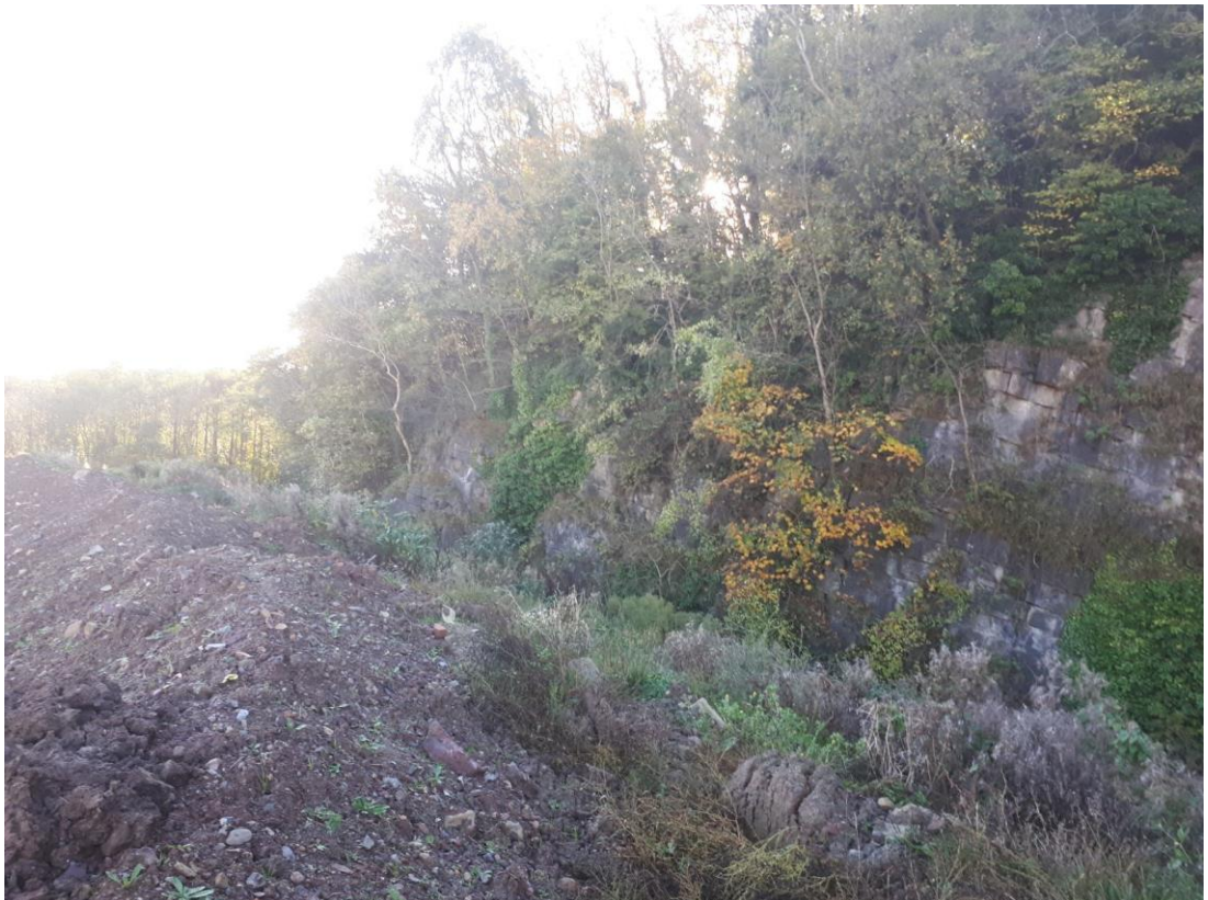
Photograph 4 – Southern sidewall showing no changes to sidewall construction – looking east
