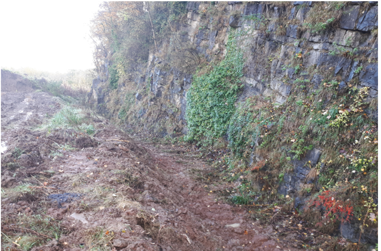
Photograph 2 – Formation surface of Southern Sidewall (east)
