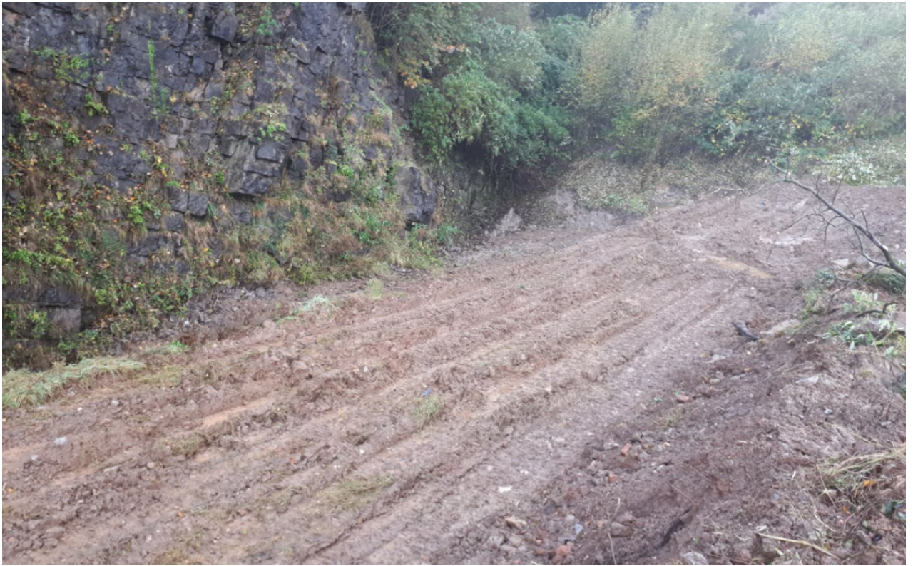
Photograph 1- Formation surface of Southern Sidewall (west)
