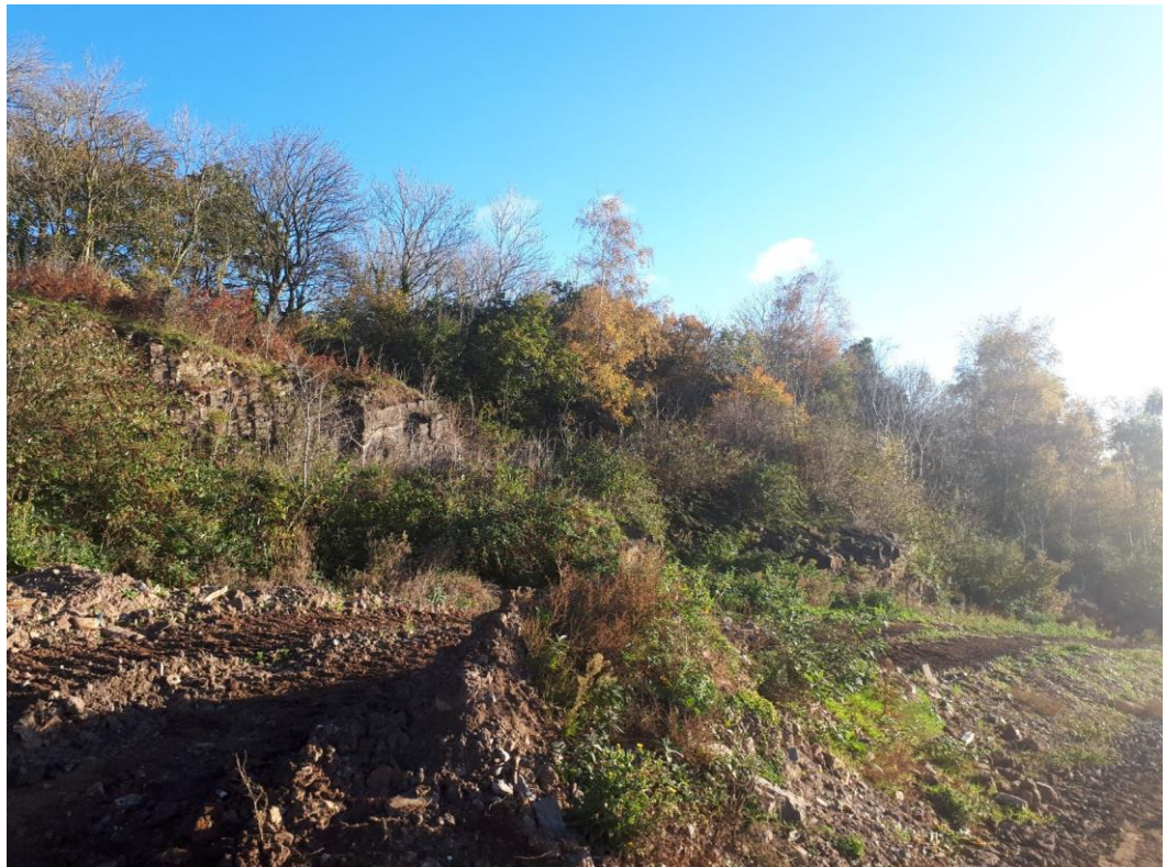
Photograph 2 – Northern sidewall showing formation for Lift 4 (surface of Lift 3) – looking east. Vegetation to be removed prior to barrier construction
