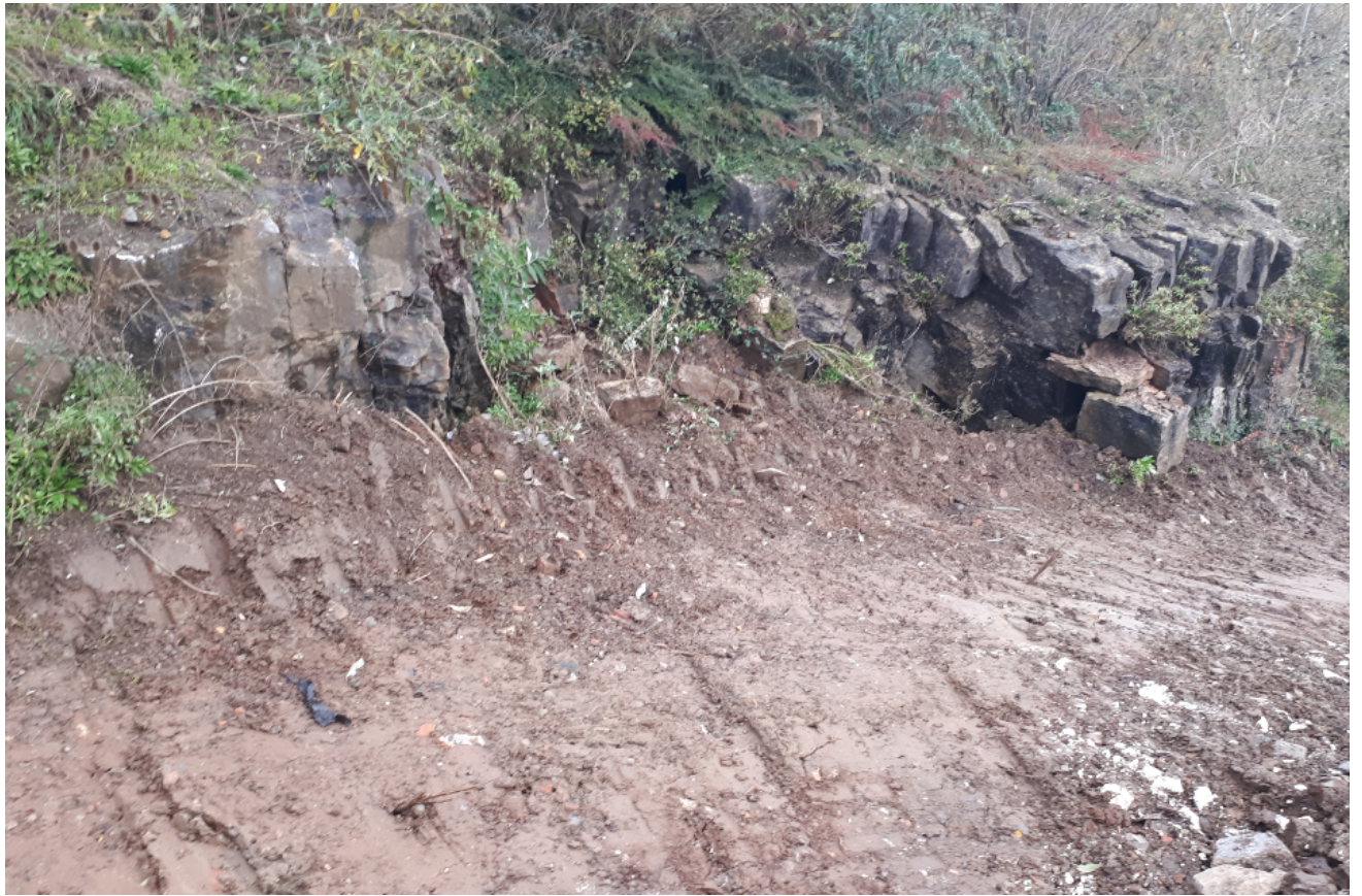
Photograph 1- Formation level of Lift 4 prior to placement of material (eastern section)
