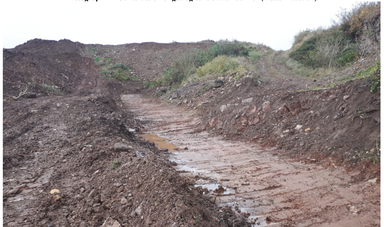
Photograph 2 – Construction of geological sidewall barrier (western section)
