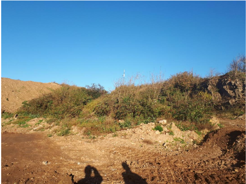
Photograph 3 – Northern sidewall showing formation for Lift 4 (surface of Lift 3) – looking west
