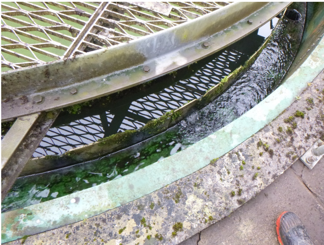
Figure 1: Final settlement tank with visible 'bubbling' coming from the base of the weir.
