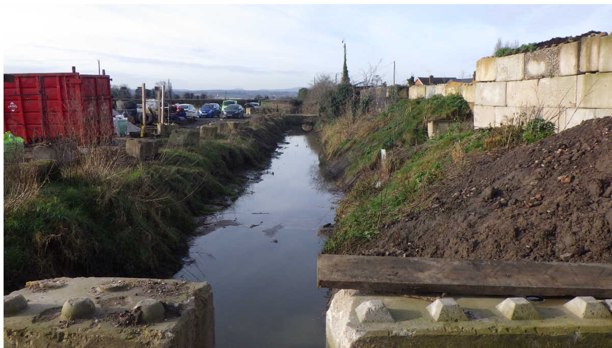
Bridge across to parking and storage.
