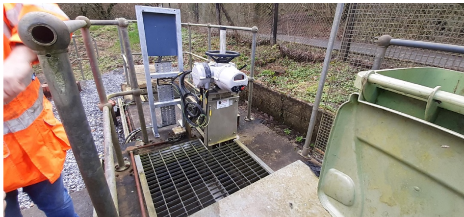
Figure 1: An image showing where storm effluent is separated from the inlet.
