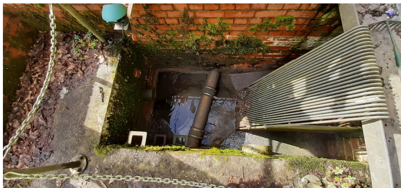
Figure 2: An image showing the chamber where final bar screening of storm effluent takes place before being discharged to the receiving watercourse.
