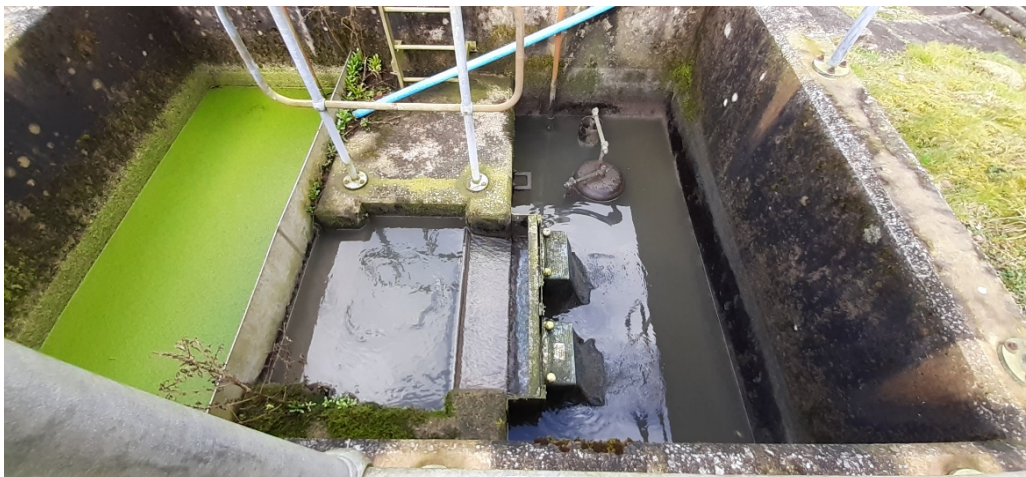
Figure 3: An image of the splitting tank.
