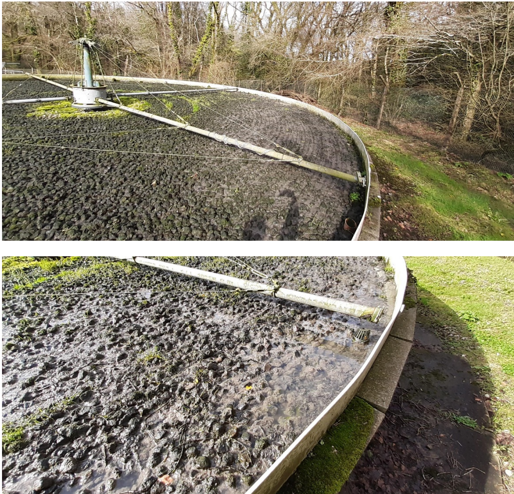
Figure 3: The top image shows the percolating filter bed with distribution arms in operation. The bottom image shows pooling on the surface of the biofilter media.
