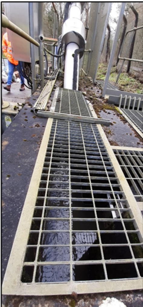
Figure 1: An image of the inlet channel with a rota screen and bar screen on the side channel.
