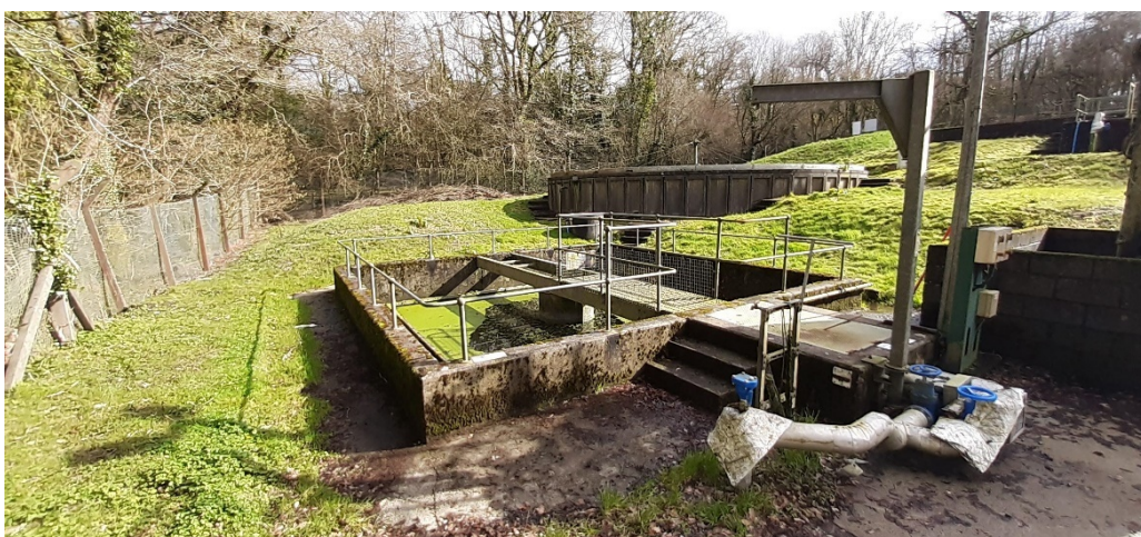
Figure 4: An image of the humus tank.
