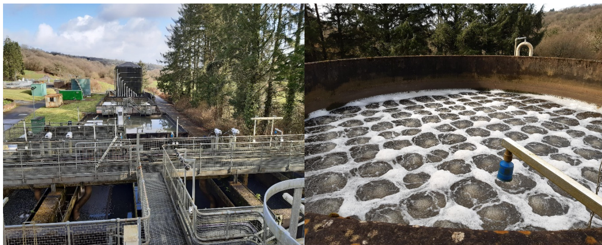
Figure 4: An image of vegetation growth on one of the percolating filter beds at the works.
