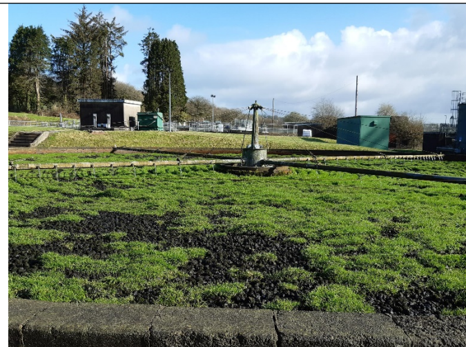
Figure 4: An image of vegetation growth on one of the percolating filter beds at the works.
