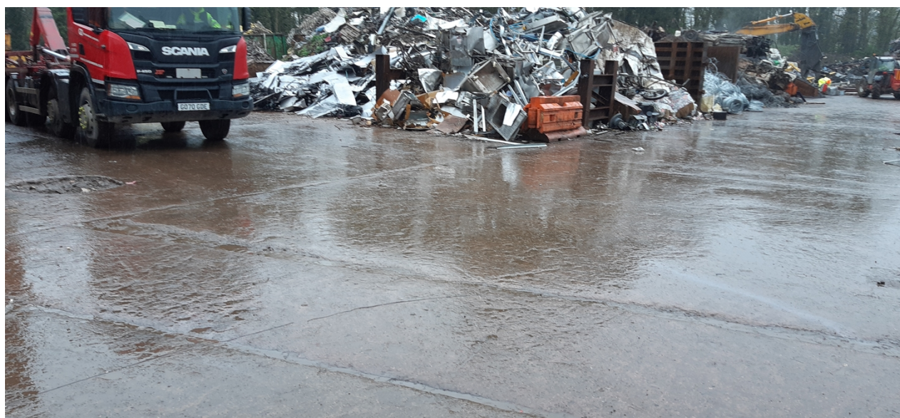
Photo 2 - Flooring infrastructure in good working order on site
