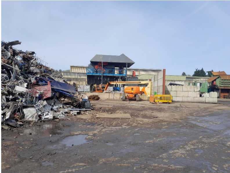
(Photograph 1 – Pre-shredder installation taking place)
