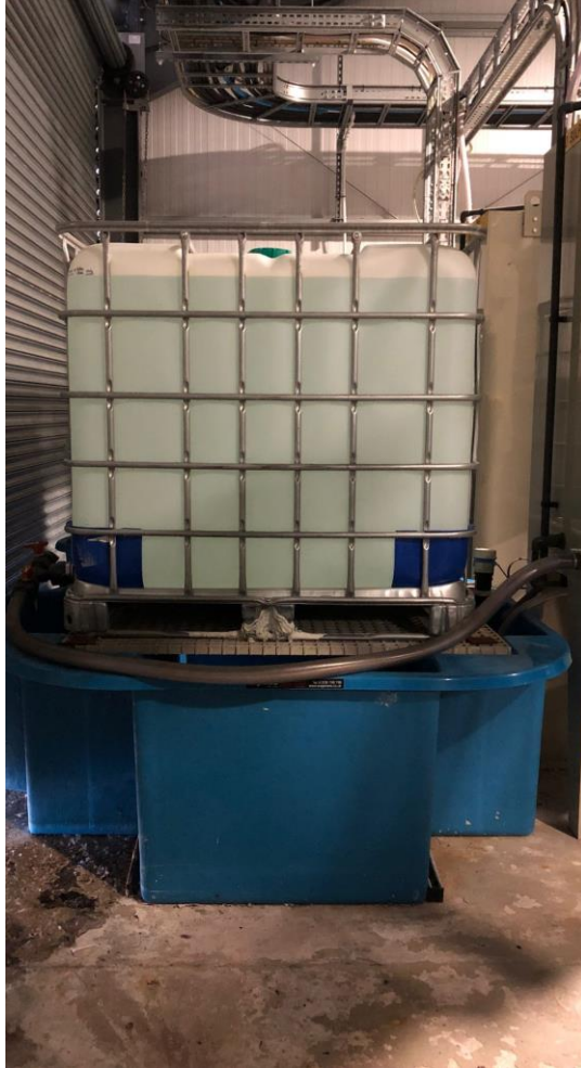
Fig 1. Bund arrangement for nutrient dosing chemicals
