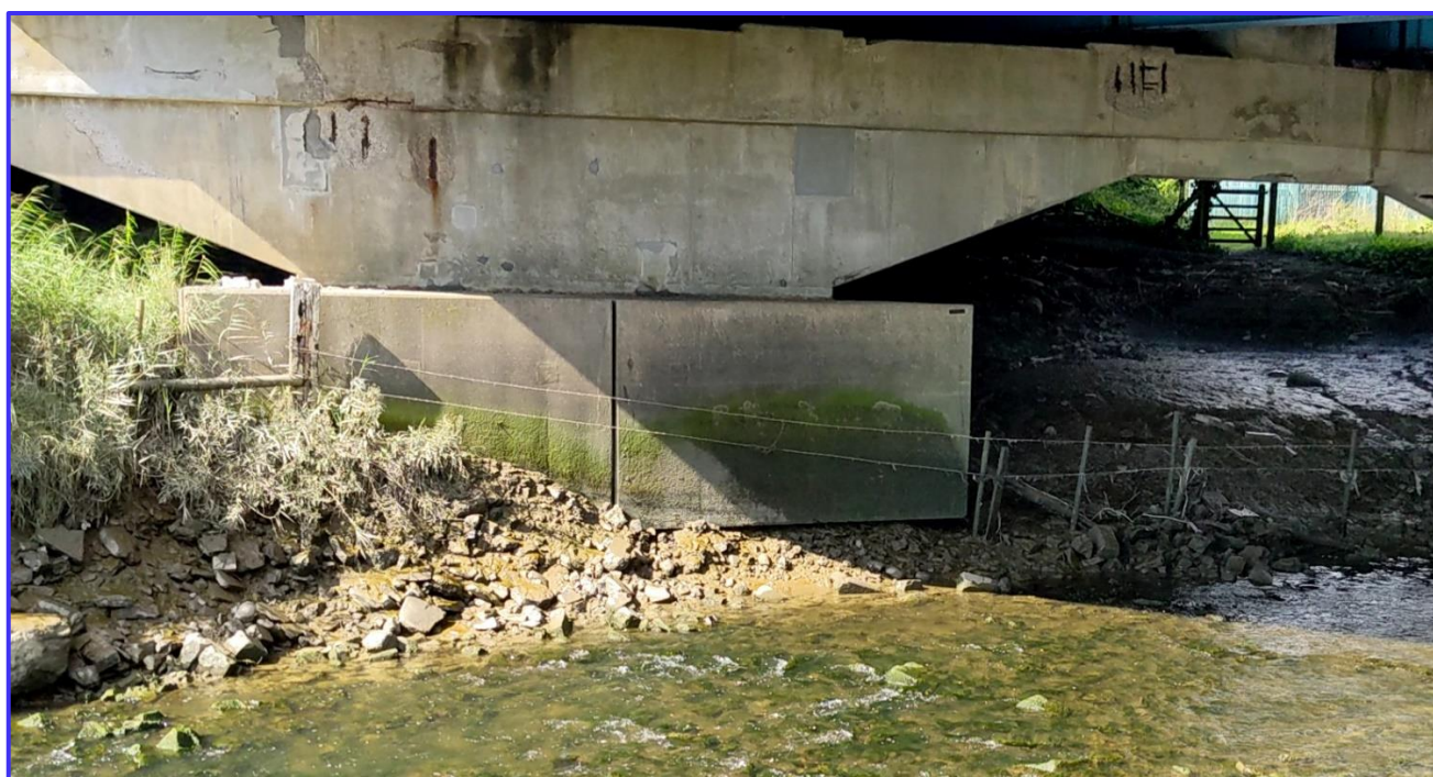
Photo 2 – Southwest pier within right-hand riverbank
