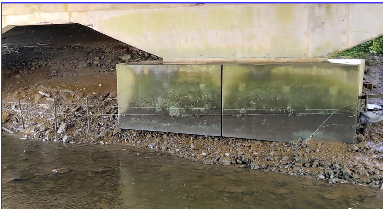
Photo 1 – Northwest pier within right-hand riverbank
