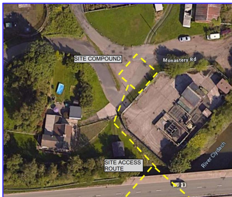
Figure 2-1 - Site compound and works access
