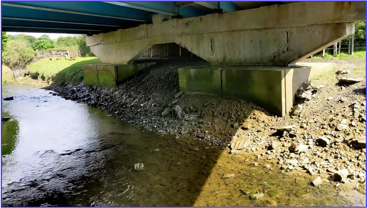
Photo 3 – Pier situated in left-hand riverbank (no associated works)
