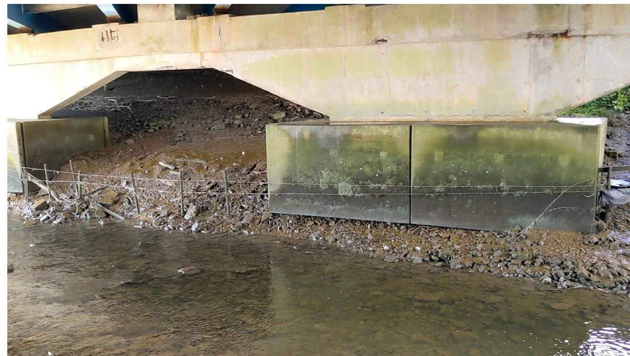
PHOTO OF NORTH WEST PIER
