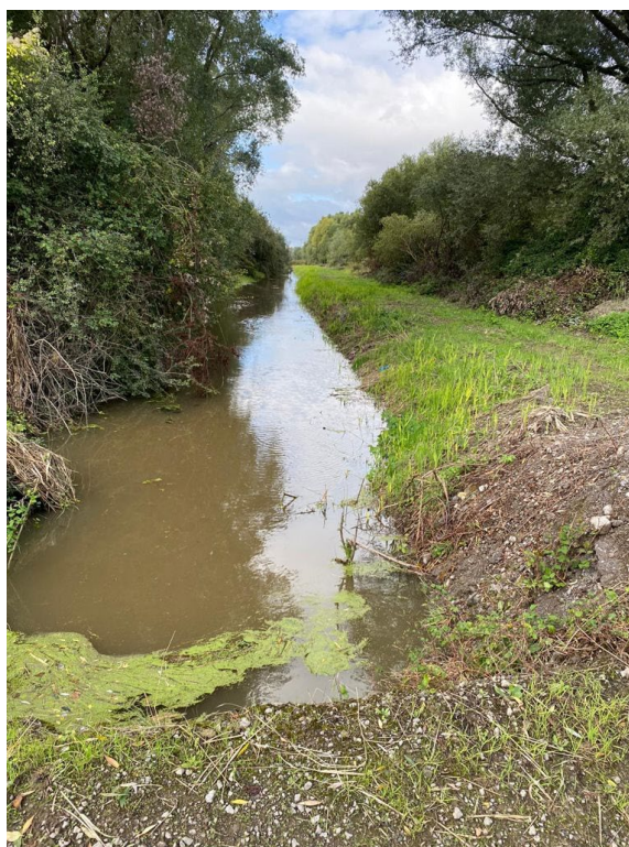
Plate 6-5 Raised surface water levels in October 2021
