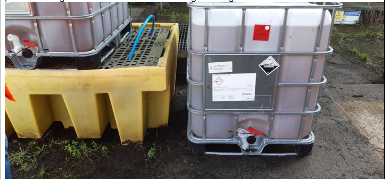
Photo showing dosing chemicals not stored on bunded area.
