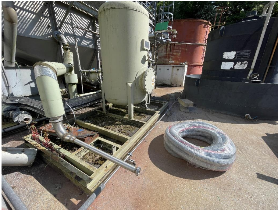
Photograph 5: Redundant ETP Main Slab Area
