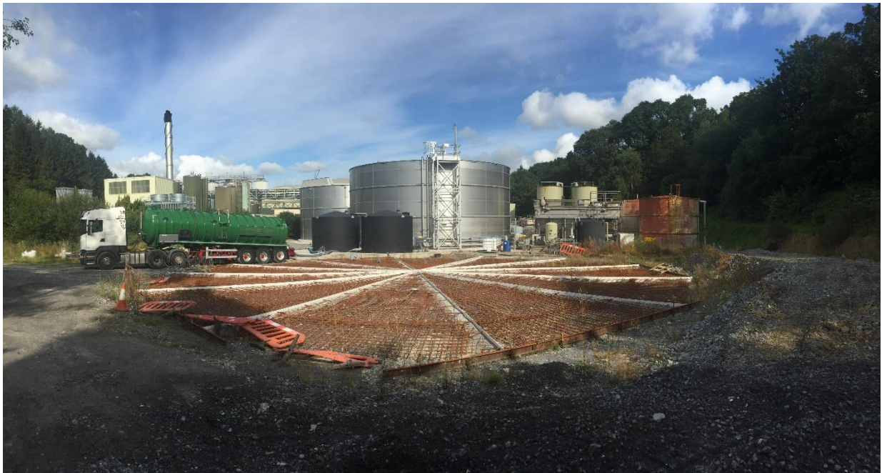
Photograph 2: New ETP and Redundant ETP
