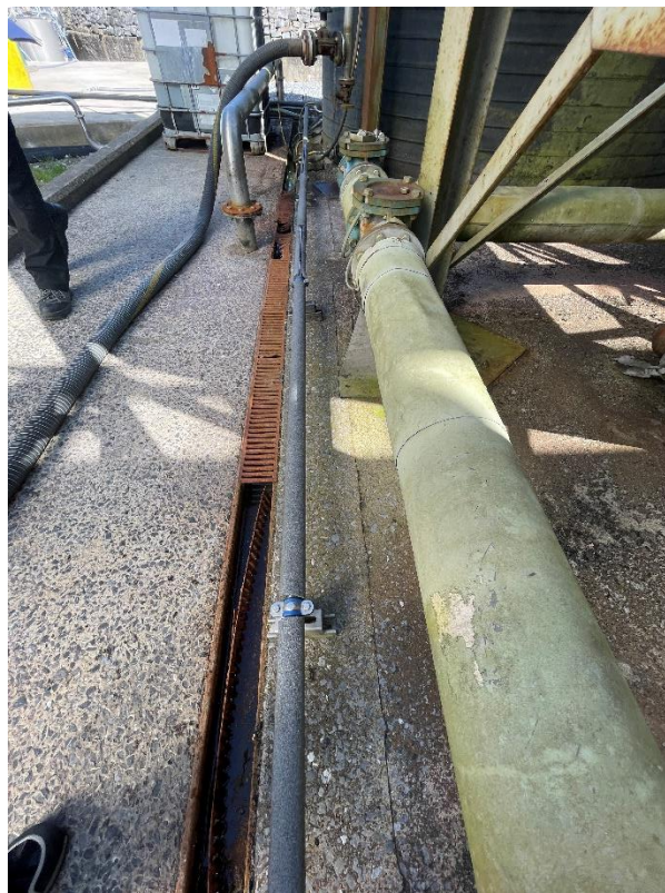
Photograph 10: Surface Water Drainage Along West Side
