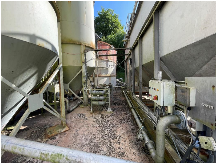
Photograph 9: Redundant ETP Slab – General View
