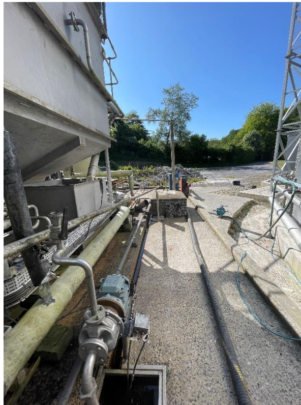
Photograph 13: Redundant ETP Slab – General View South East
