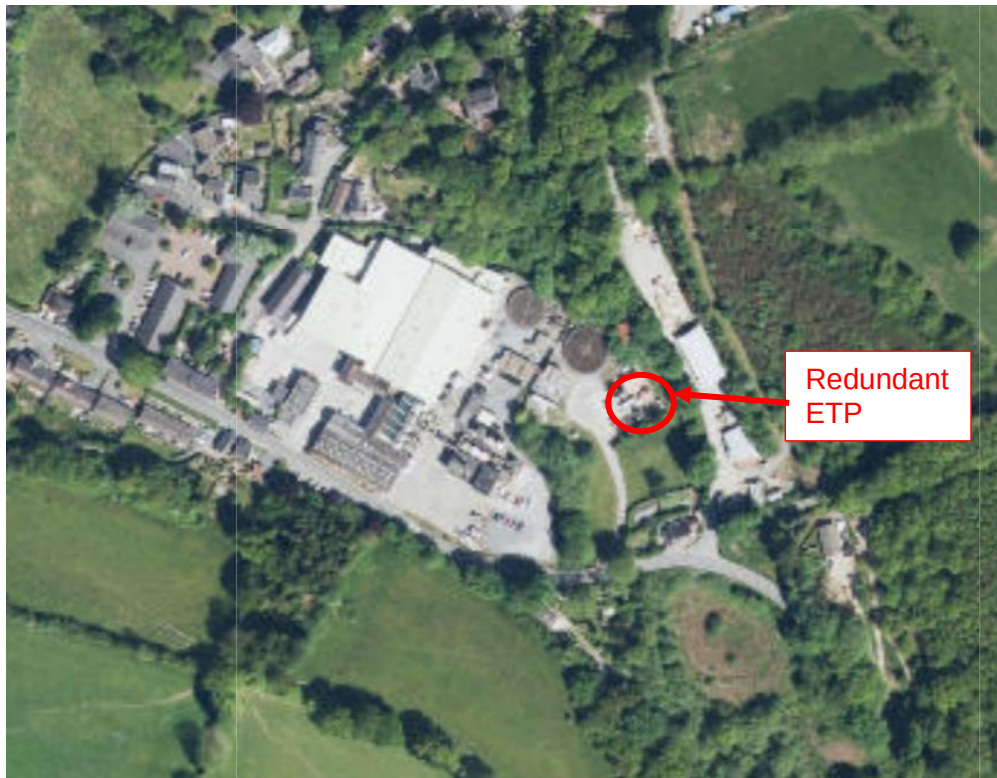
Photograph 1: Aerial Photo of Pre-Developed Site
