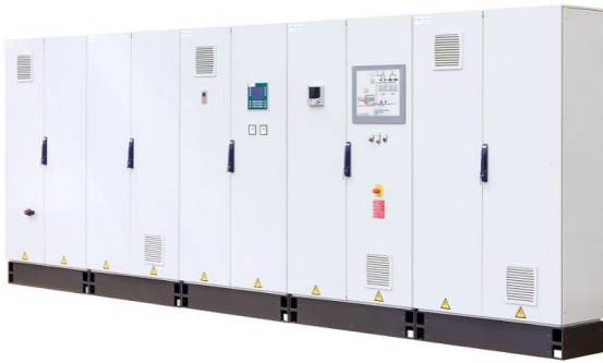
Control panel with touch panel
