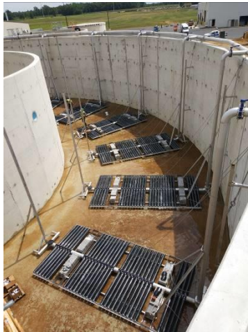
Liftable aeration grids installed
