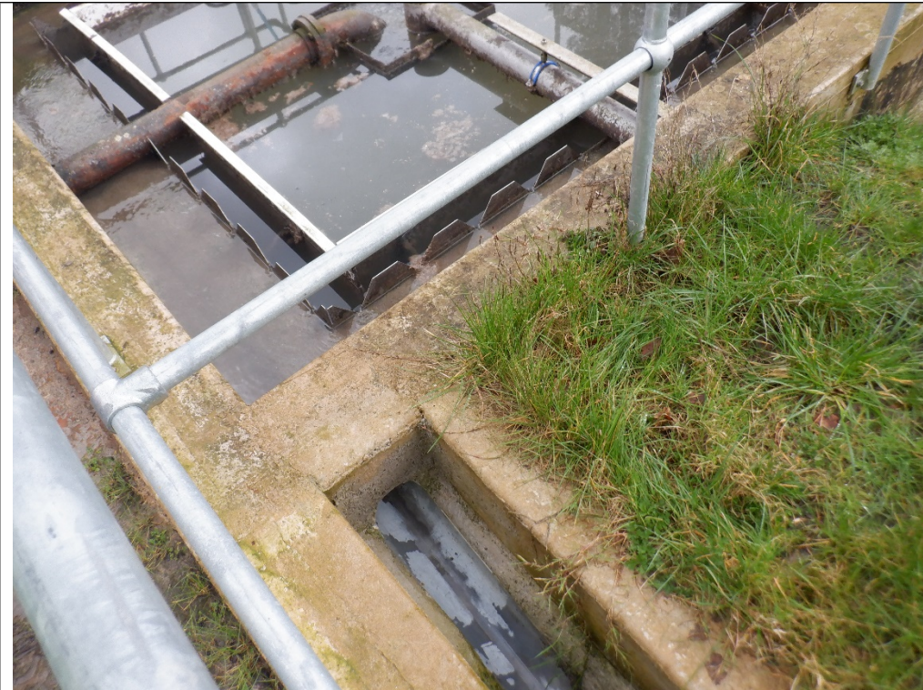
Figure 2 Second overflow pipe on the primary tank with no EDM monitor on
