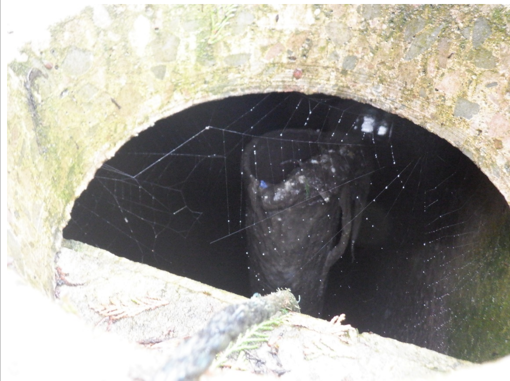
Figure 2 Second overflow pipe on the primary tank with no EDM monitor on
