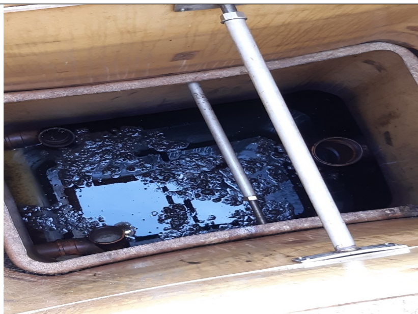
Figure 7 Final effluent chamber
