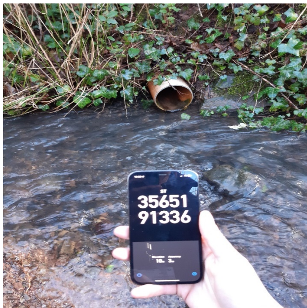
Figure 5 Discharge point for the system (shown as consent point in the permit)
