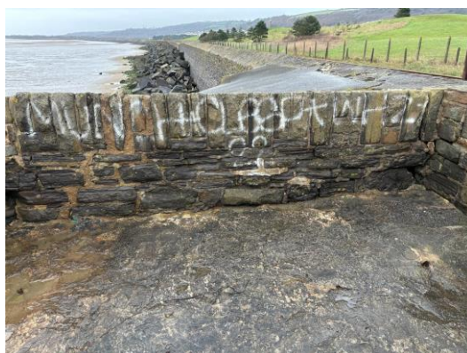
Suitable anchor points can be drilled into concrete to set up SSOW
