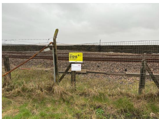
Remove fence panel for access and replace when complete.
