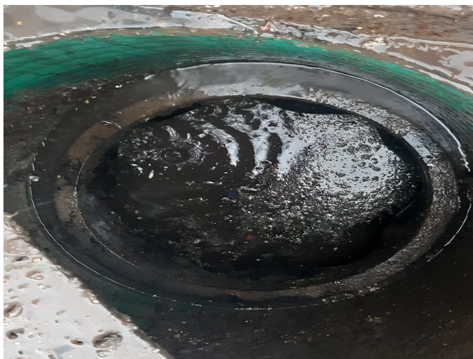
Figure 5: Final interceptor chamber
