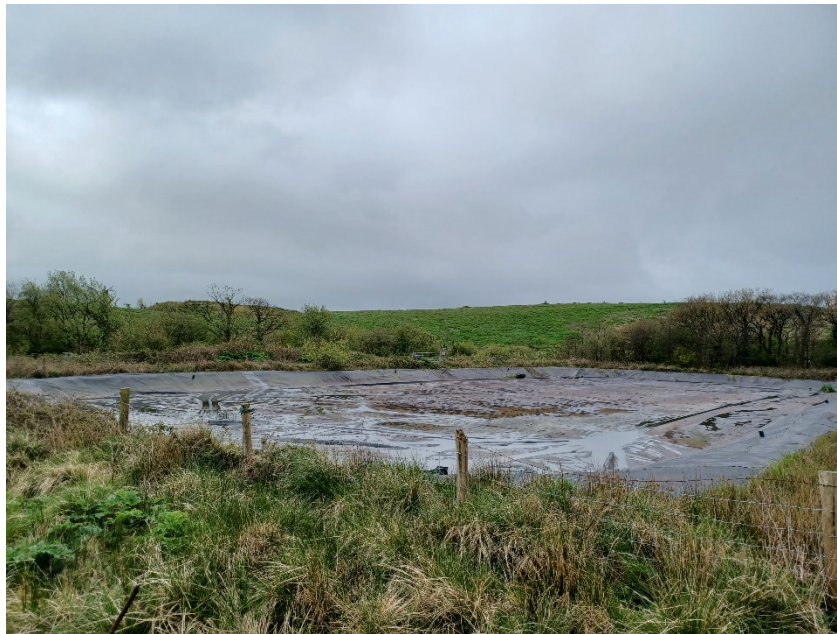
Image 1: Nantycaws Landfill Leachate Holding Lagoon
