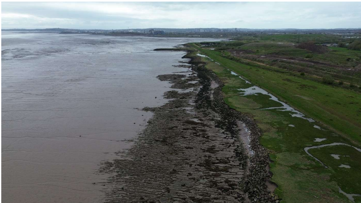
Photographs 1 to 2 showing main areas of work.
