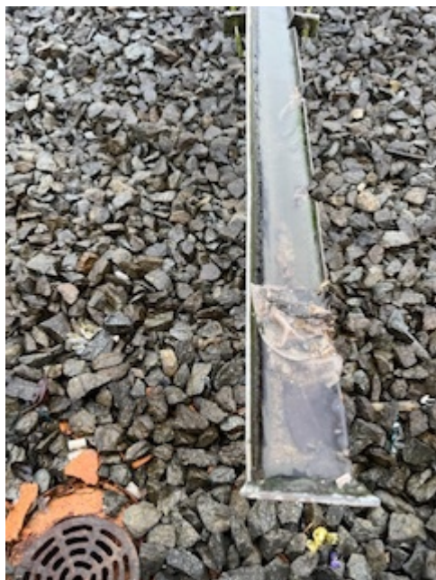
Image 4, debris on distribution arm
