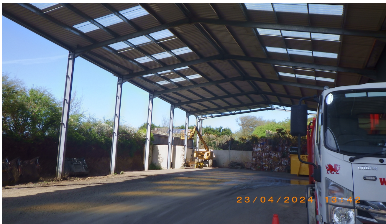
Photograph showing new roof in yard area
