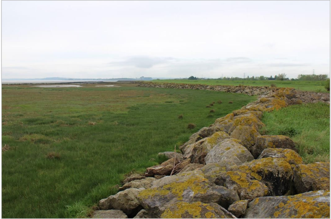
Photograph 9: Rock armour wall protecting alluvial silt deposits. Looking southeast. Looking southwest.
