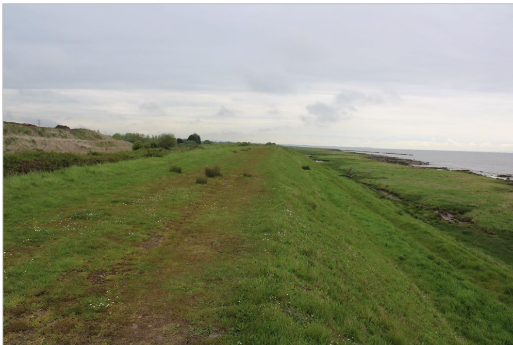
Photograph 6: Showing southern end of 20 th century sea wharf. Looking northeast.
