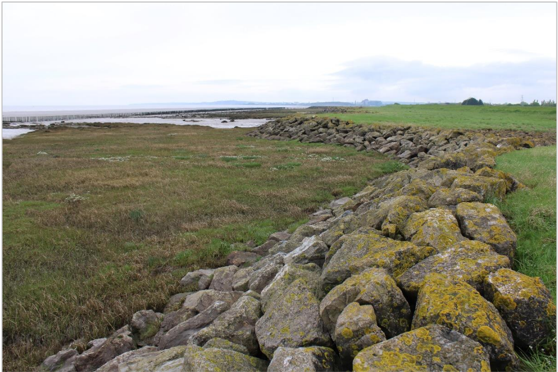
Photograph 2: Showing former coastal defence made of large boulders with pasture above and saltmarsh beneath. Rumney Great Wharf (Cadw: GM474) stands to the rear right.
