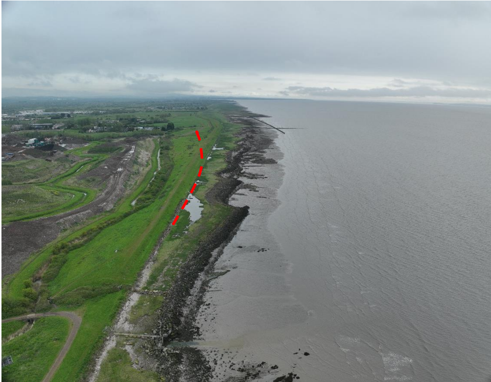
Photograph 4: Highlighting in red the 'Relict Seawall Rumney Great Wharf' scheduled monument (Cadw: GM474) behind the modern sea defences. Looking northeast.
