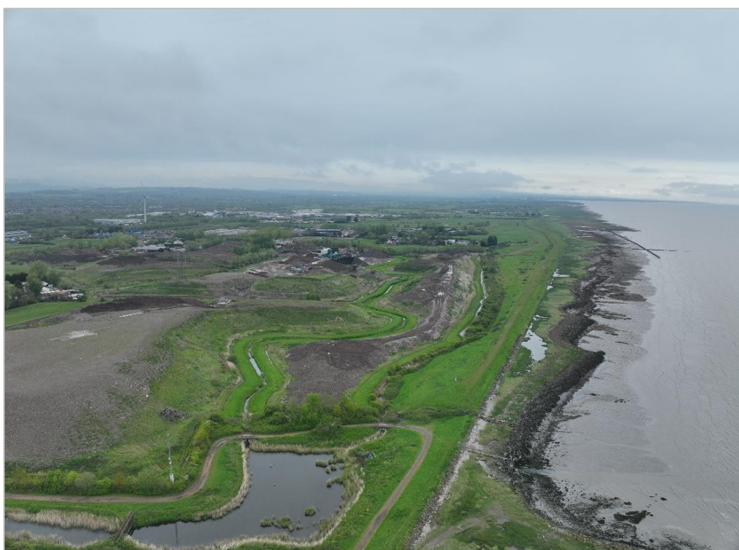
Photograph 7: Alluvial plains extending beyond the sea defences. Looking north.
