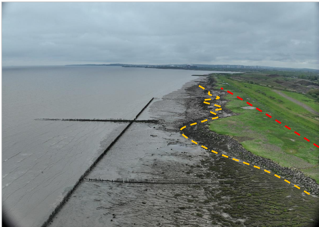
Photograph 8: Showing 20 th century wharf outlined in red and the modern rock armour wall in yellow. Looking southwest.
