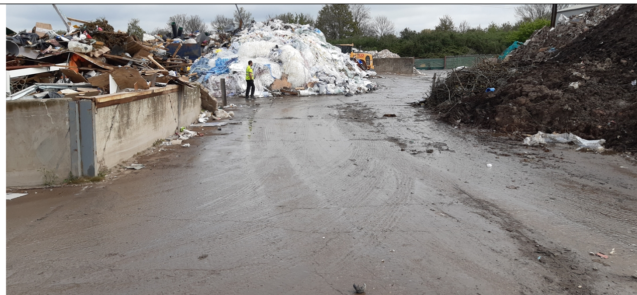
Photo 3 - Improved areas of flooring infrastructure
