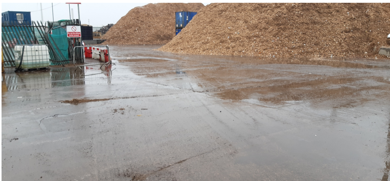
Photo 2 - Housekeeping and flooring infrastructure at SWWP Ltd, Alexandra Docks
